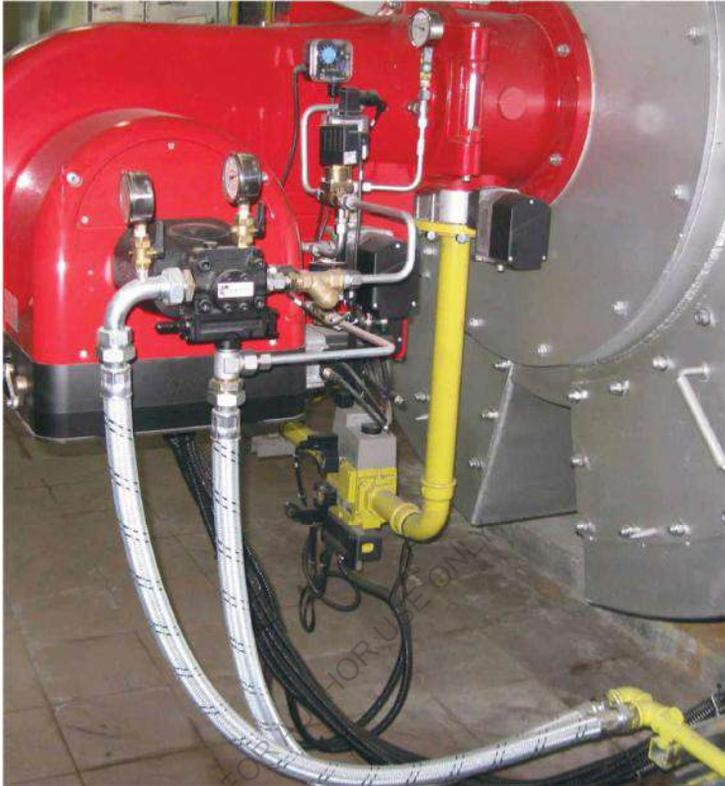
**Figure 1-1 - 2**, - the figure shows an automatic fuel system module for an industrial boiler with a capacity of 10 tonnes of steam per hour.
