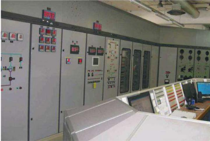
**Figure 1-2,** - the figure shows the central control and monitoring panel for a group of industrial boilers, each with a capacity of 10 tonnes of steam per hour.
