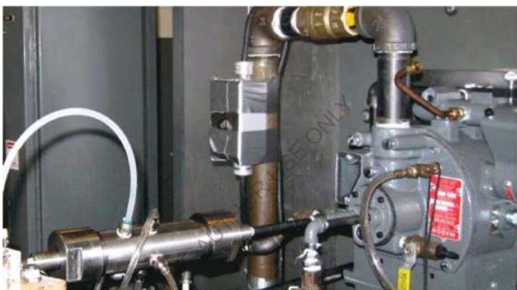
The use of a device with an operating diameter of 25 mm, designed to form an emulsion of diesel 2 and tap water in a ratio of 70% diesel to 30% water in a modern boiler.
