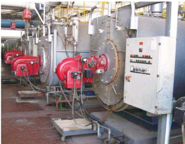
**Figure 1-1**, - shows the engine room with industrial boilers installed, each with a capacity of 10 tonnes of steam per hour.
